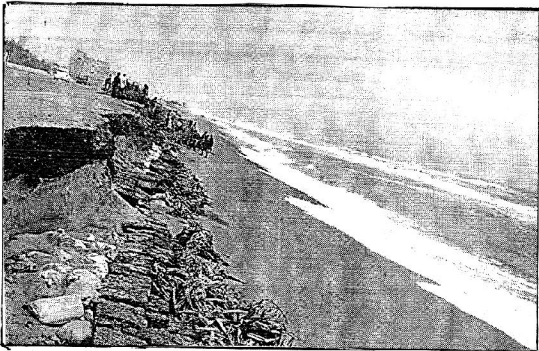
Fig.4. Damaged public road of Puri coastal belt
