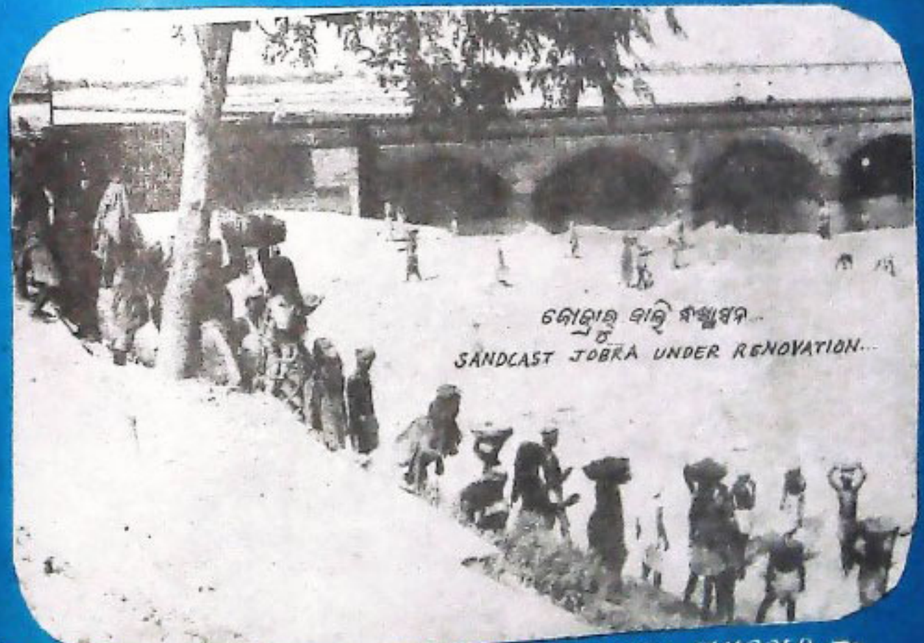
ଦଳେଇପାଈର ମରାମତି - DALEIGHAI BREACH BEING PLUGGED...
